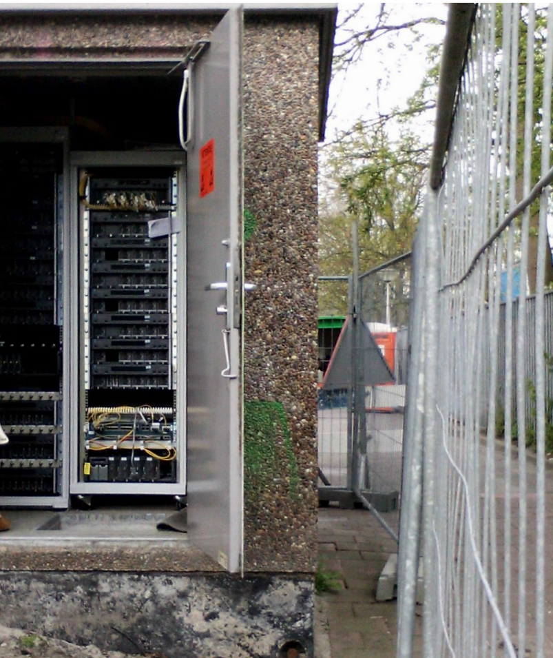
Figure 2 Threshold of a few decimeters above ground within substations
