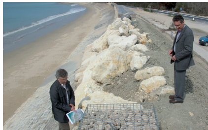
Experts inspect emergency repair work carried out following Cyclone Xynthia. Copyright: Rémy Tourment
