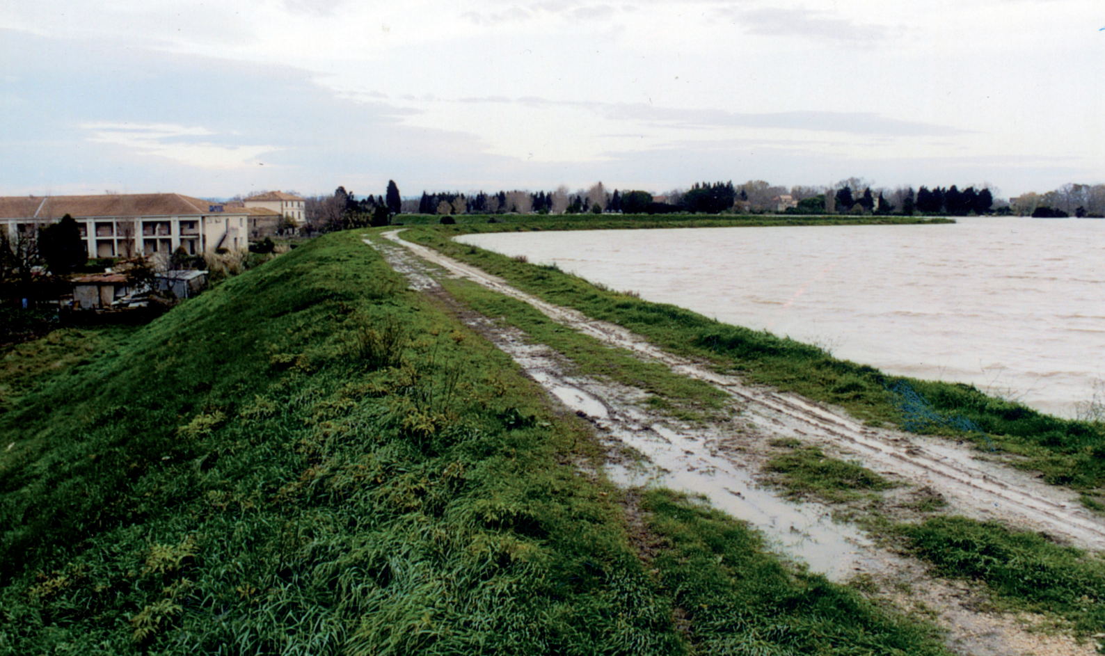
Flood of the River Rhone in December 2003 in Fourques (Gard, South France). The dykes protect the town. Copyright: Paul Royet
