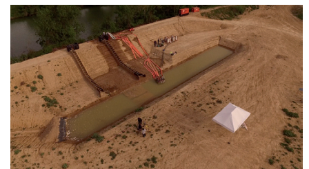
An aerial view of the soil-lime experimental embankment under construction. DigueElite project. Copyright: Dronimages
