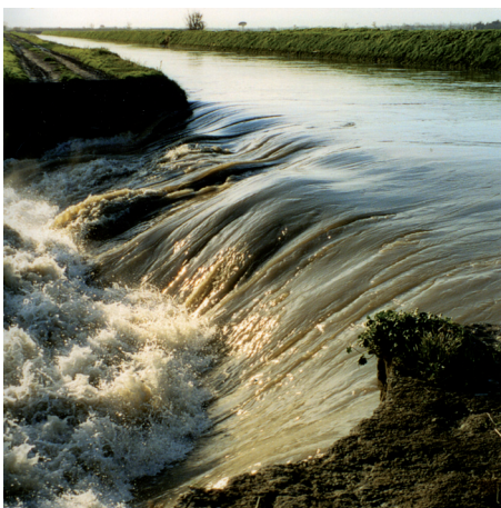
Breach on the Vigueirat dykes in December 2003 Copyright: Rémy Tourment
