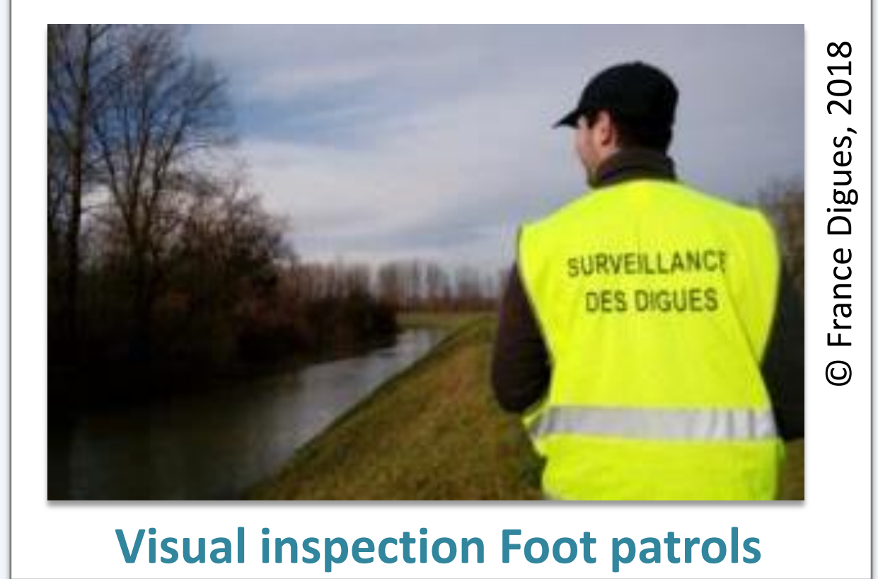
Visual inspection Foot patrols
