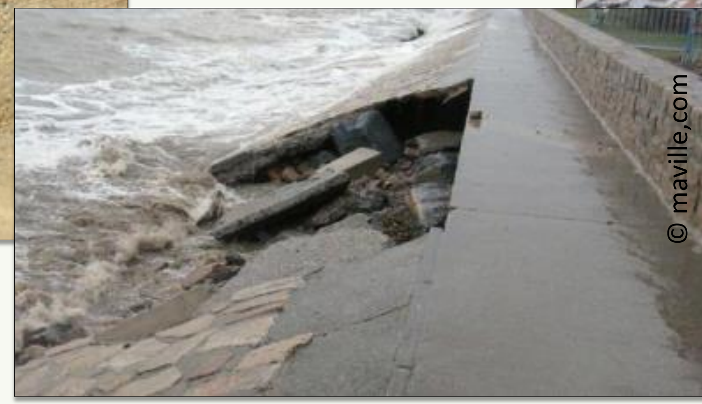
Damaged masonry seawall
